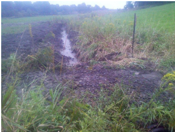
Culvert newly repaired at Heldeberg Airport in East Berne.
