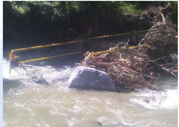
The bridge washed downstream from C7B near Maple Inn, East Berne.
