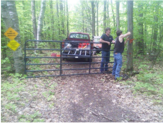
Karl Pritchard and VP Ron Shultes install a new gate on the trail.
