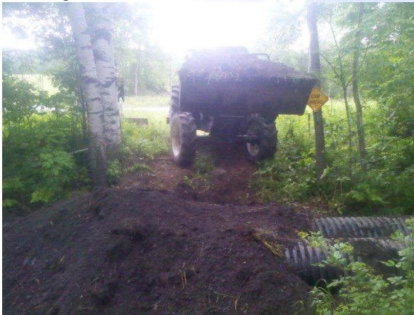
A load of dirt is dropped on culvert tubes earlier this summer.
