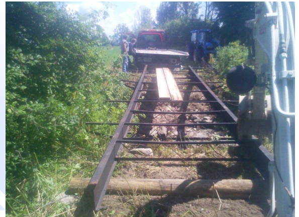
In July, a new bridge frame is lowered into position along C7B in Knox.
